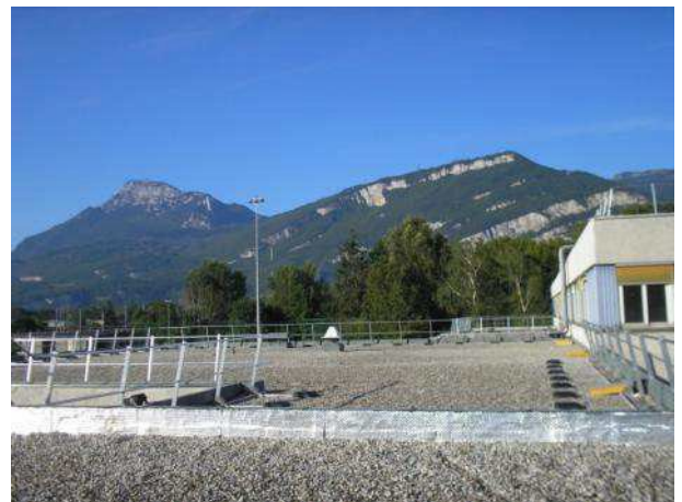
Photo 2 - Gravel terrace with retention system
