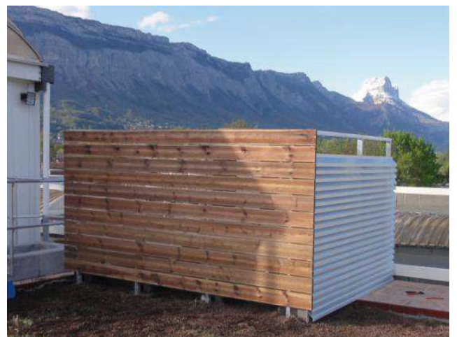
Example of a wooden slat cladding
